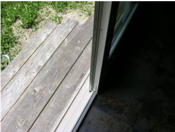
Photo 4-1 Temporary landing and steps off the rear sliding glass door
