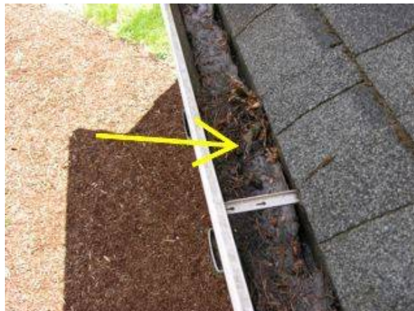
Photo 5-2 Debris in the gutters
