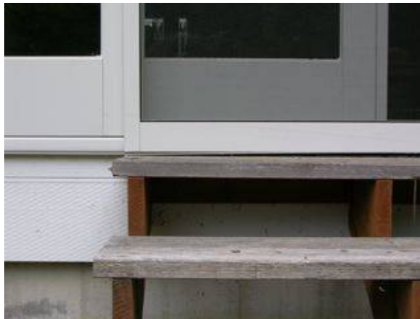
Photo 4-2 Temporary landing and steps off the rear sliding glass door
