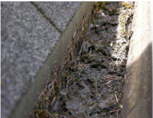
Photo 5-1 Debris buildup in the gutters
