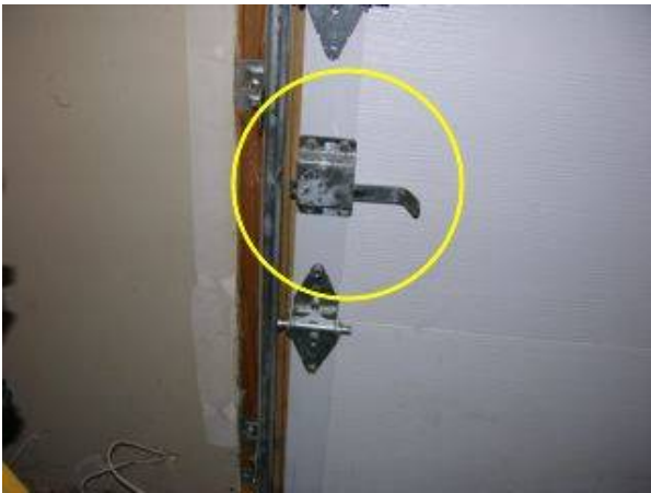
Photo 13-1 Garage door locks present with garage door openers. All three doors
