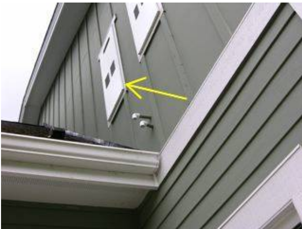
Photo 26-1 Unable to remove the panel on this water heater.
