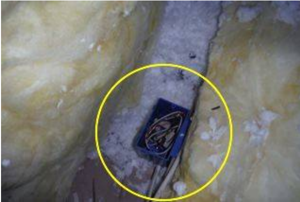
Photo 14-1 Open box in the attic
