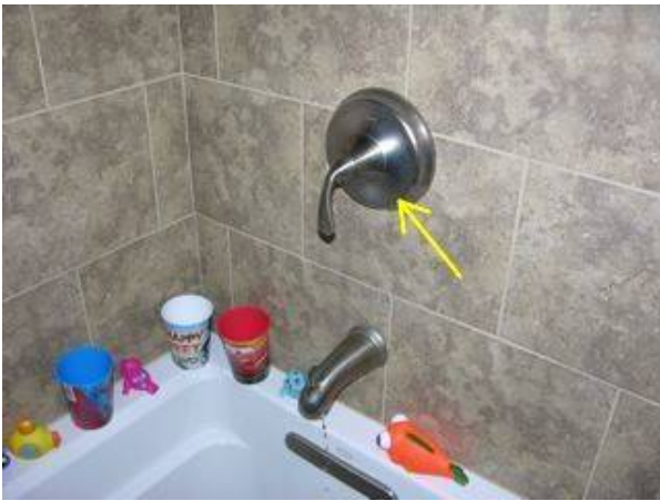
Photo 37-1 Direction of hot and cold reversed.
